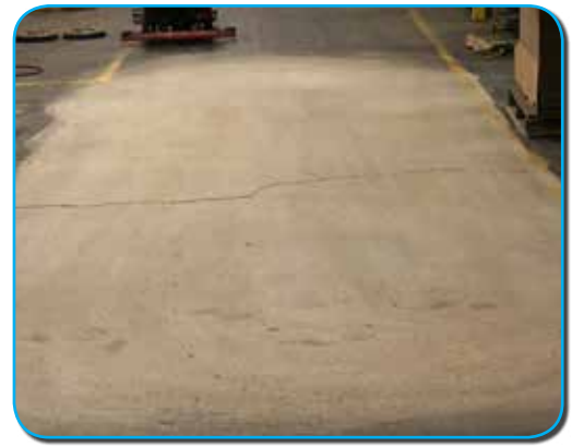
FIGURE 2-A: AFTER 100 GRIT CONCRETE PREP TOOL. YOU WILL NOTICE ANY DIPS IN THE FLOOR THAT MIGHT NEED ANOTHER PASS OR TWO.
