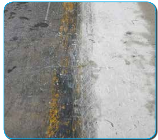
FIGURE 2-B: UNIFORM WHITENING ON THE CONCRETE WILL BE VERY NOTICEABLE. IF NOT - CONTINUE PROCESS TILL FLOOR IS UNIFORM.
