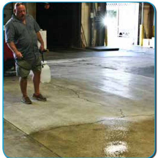
FIGURE 3-B: LAYING DOWN DENSIFIER WITH SPRAY TOOL.
