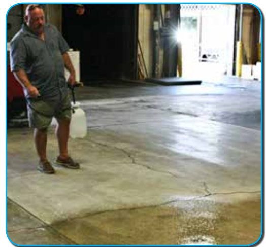
FIGURE 5-A: LAYING DOWN DENSIFIER WITH SPRAY TOOL.
